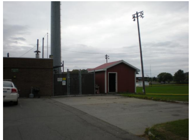
Well Maintained Site
